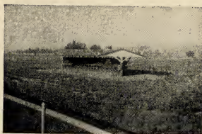
One of forty feed sheds.
