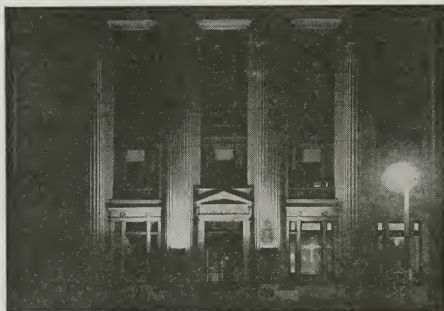
LDS. CHURCH ADMINISTRATION BUILDING
