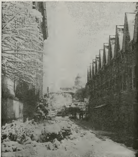
—Photograph by James E. Asper AN UNUSUAL VIEW OF THE STATE CAPITOL BUILDING
