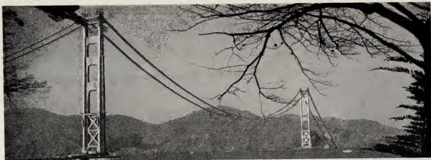
GOLDEN GATE BRIDGE LOOKING TOWARD THE MARINE SHORE FROM SAN FRANCISCO, SHOWING THE WORLD'S LONGEST SINGLE SPAN, 4,200 FEET.
