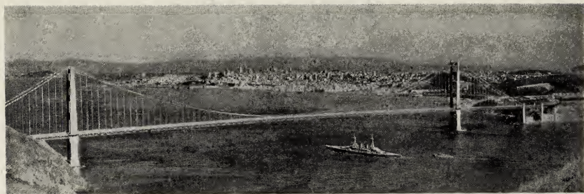
AS THE GOLDEN GATE BRIDGE WILL LOOK WHEN OPENED TO TRAFFIC, MARCH 1, 1937.
