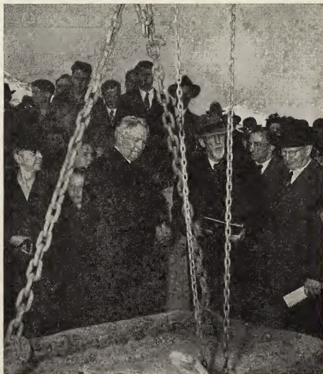
Laying the cornerstone of the "This is the Place" monument. Left, foreground, President David O. McKay; center, President George Albert Smith; extreme right, Elder John D. Giles.
