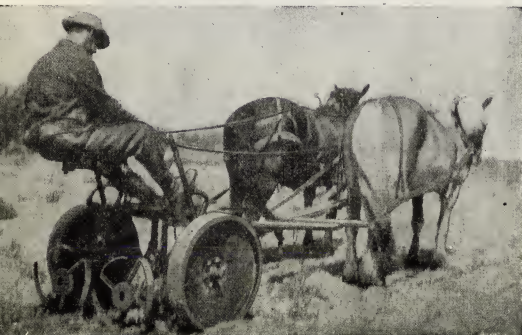
This new machine, the Dixie Thinner, almost entirely eliminates the necessity of thinning by hand. The twin whirling knives at the rear cut out the excess beets.
