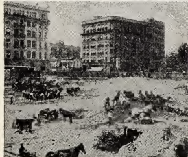
No high powered tractors, bulldozers, trucks or steamshovels grace this landscape as excavation begins.
